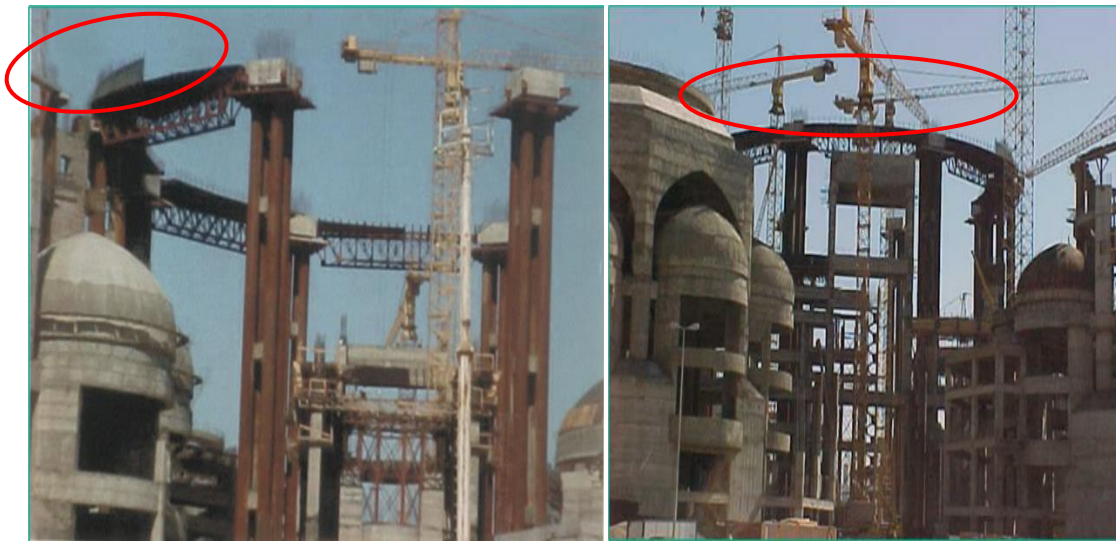
Figure 5: the construction stages of the ring beam at the height of 60 m above ground level.
